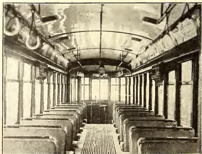
REMODELED INTERIOR, SHOWING SANITARY STRAPS
